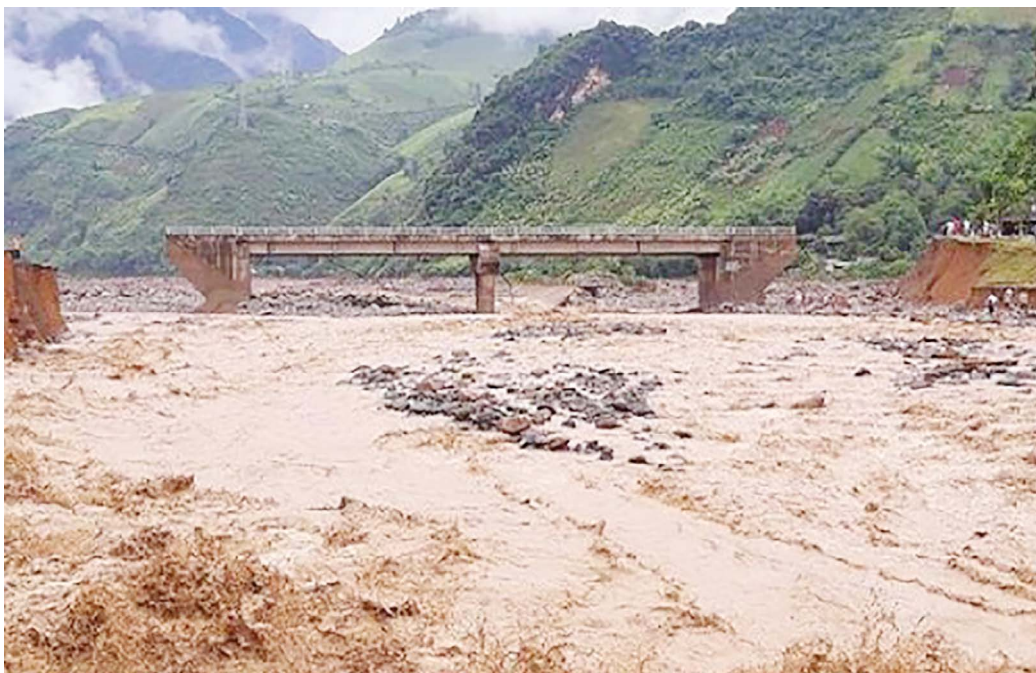
Figure 6. Nam Pam bridge destroyed by flash flood
